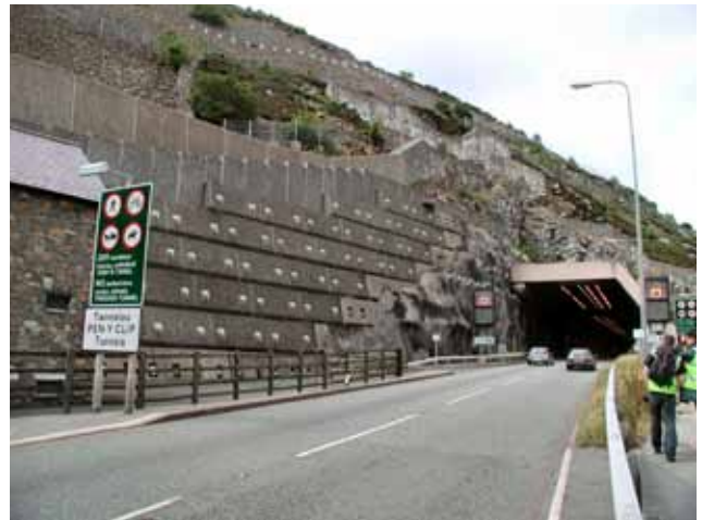
Multiple rockfall protection systems installed near the Pen-Y-Clip tunnel on the A55 North Wales Expressway, United Kingdom. (Photograph: David Giles, University of Portsmouth, United Kingdom)
